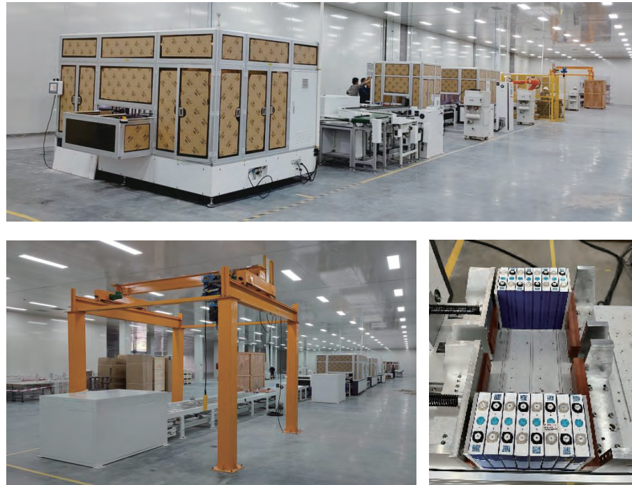
Battery module pack assembly line
